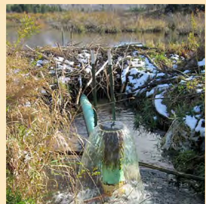
Figure 4. A pond leveler can be used to maintain water levels allowing beavers to remain on location.
