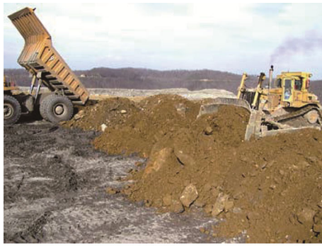
(a) Placement of brown topsoil up to 1.5 m in depth
