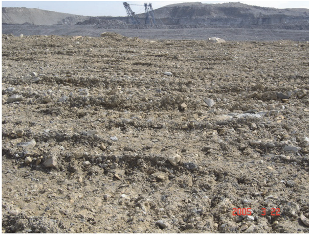
Fig. 2. Brown sandstone compacted plots before planting with trees.
