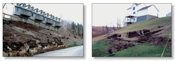
Steep slopes around buildings can cause instability, erosion, and landslides, all of which require complex and expensive corrections. Soil and water movement will often result in building foundation problems, such as cracking and bowing, and can damage other structures, such as concrete or block walls.
