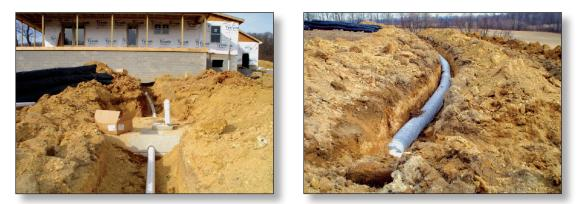
On-site septic systems require a septic tank and a drain field, where wastewater is released slowly into the soil for treatment.
