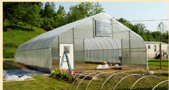
Figure 4. Gable vent in a high tunnel end wall. (Photo credit B.E. Liedl)
