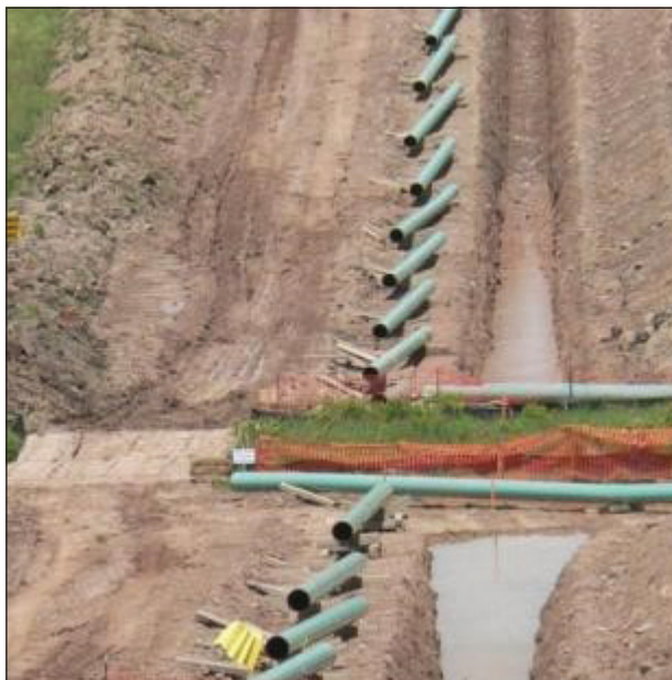
A natural gas pipeline during construction.
