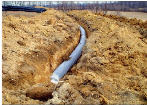
*On-site septic systems require a septic tank and a drain field, where wastewater is released slowly into the soil for treatment.*
